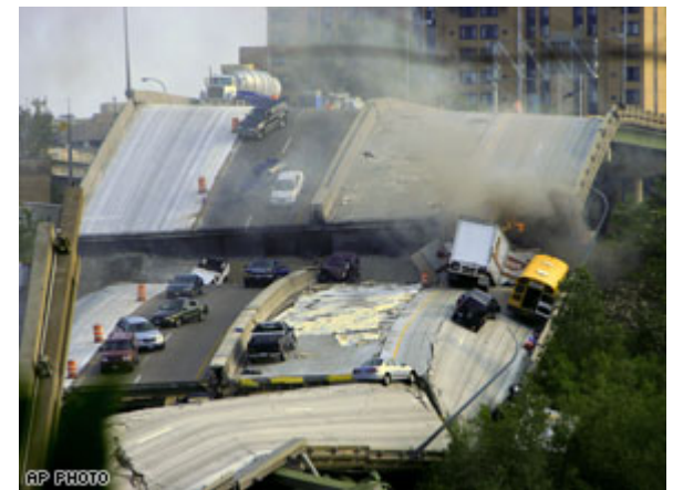
Minneapolis Bridge Collapse
