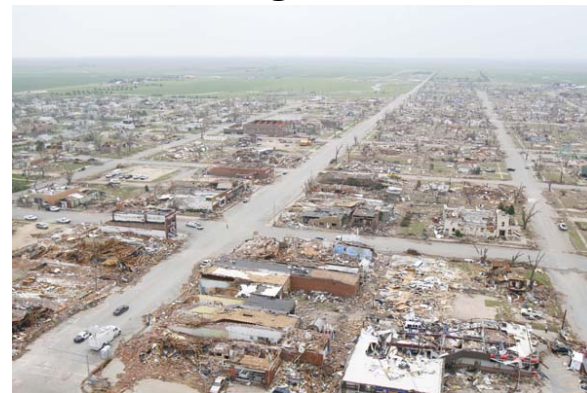
Greensburg KS Tornado
