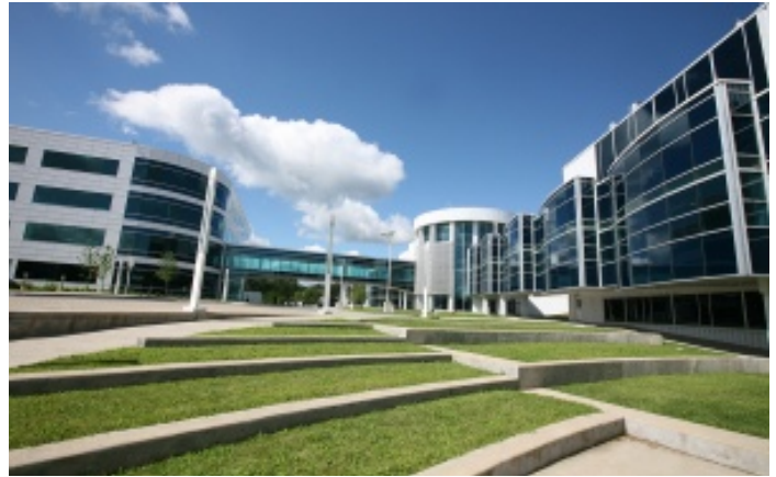
ITS's Albany Data Center
