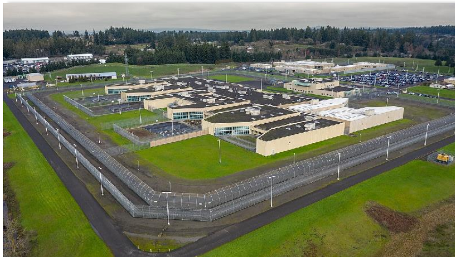
Coffee Creek Correctional Facility, Wilsonville Oregon
